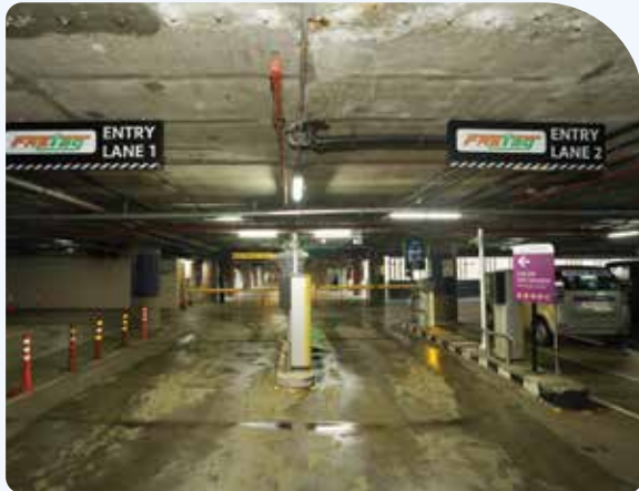
Parking guidance system for passengers An advanced parking guidance system at Terminal 2 provides real-time information on available parking spaces, streamlining entry procedures and optimising the parking experience at MIAL.
